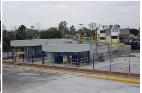
WWTP general view
